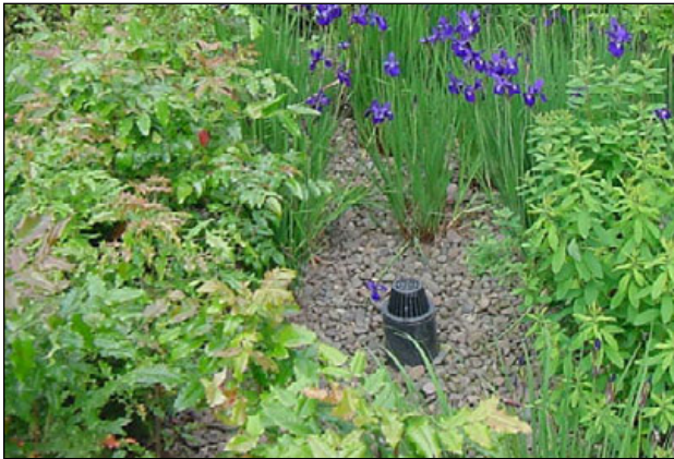
Figure C-31. A small-scale overflow stand pipe.
