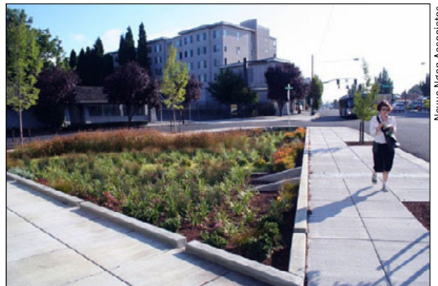
Figure C-6. A raised curb alerts pedestrians of a grade change in the rain garden.
