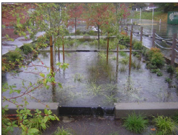
Figure C-26. Concrete check dam with an adjustable weir.
