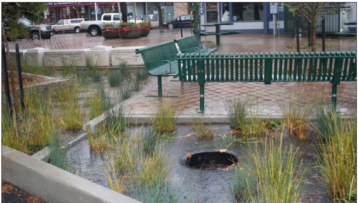
Figure C-33. A weir retains stormwater to a 8" depth before overflowing into the storm system.
