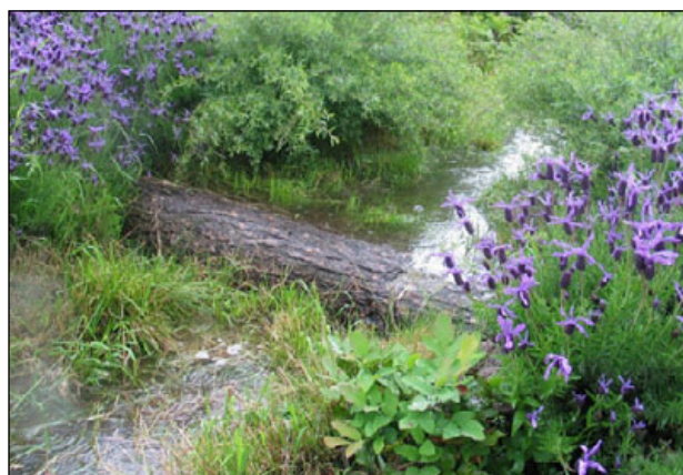
Figure C-29. Log check dam.
