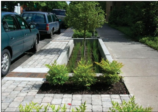
Figure C-2. A street using stormwater planters. Notice the 3-foot egress zone between the parked cars and the edge of the stormwater planter.
