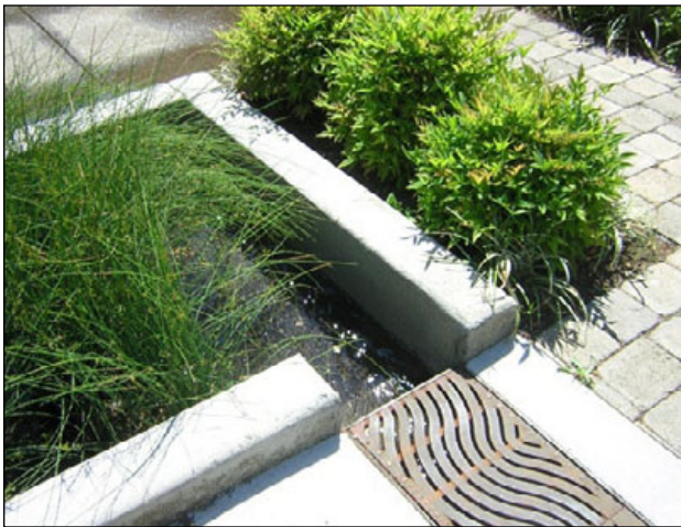
Figure C-24. Sediment forebay in a street planter.
