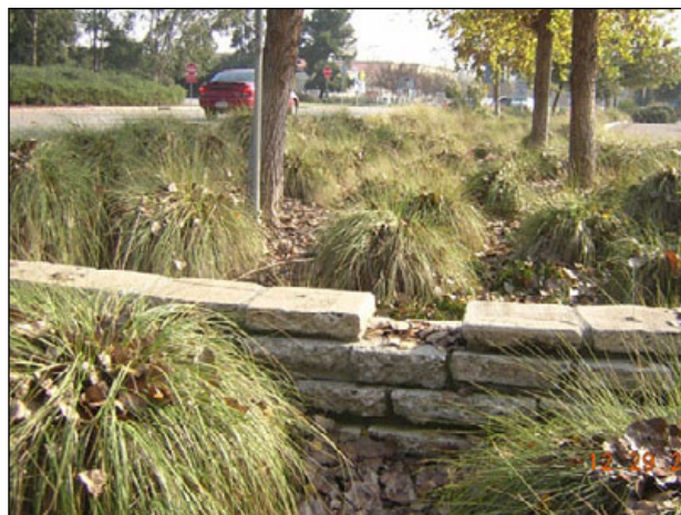
Figure C-27. Stacked concrete check dam.
