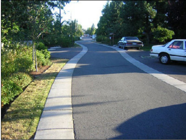
Figure C-11. Curbless street allows for sheet flow of stormwater.
