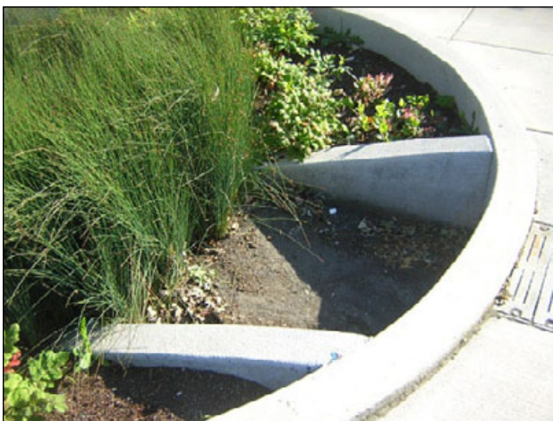
Figure C-25. Sediment forebay in a street infiltration garden.
